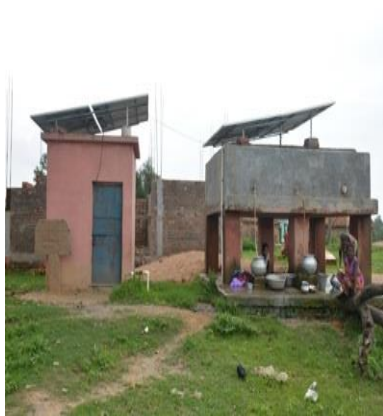
DEEP BORE WITH SOLAR POWERED SUBMERSIBLE PUMP M&A
