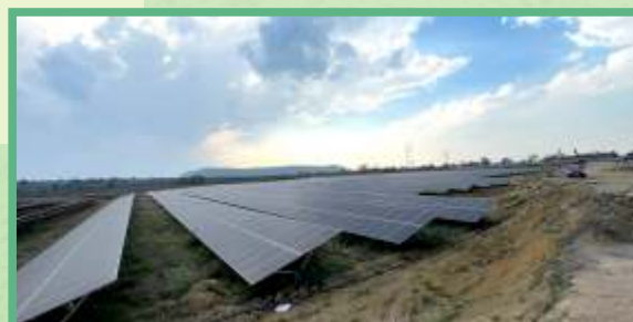
View of 4MW solar panel at Giridih Area
