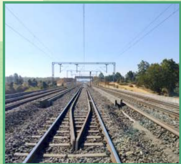
View of Tori-Shivpur 3rd rail line
