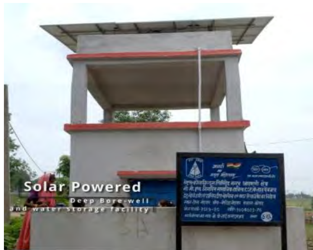
Solar Power operated Deep Bore well
