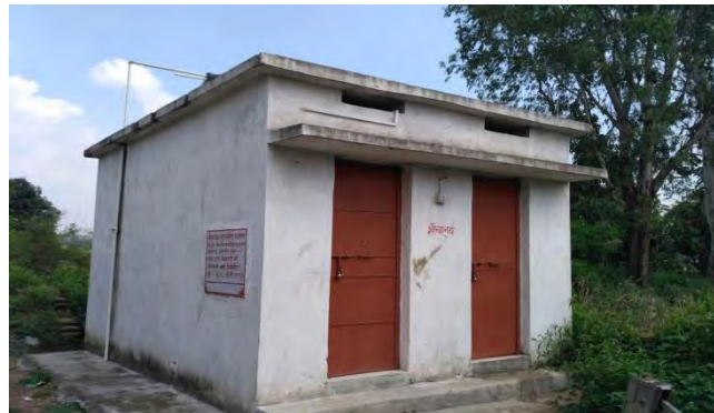
Toilet Constructed under CSR
