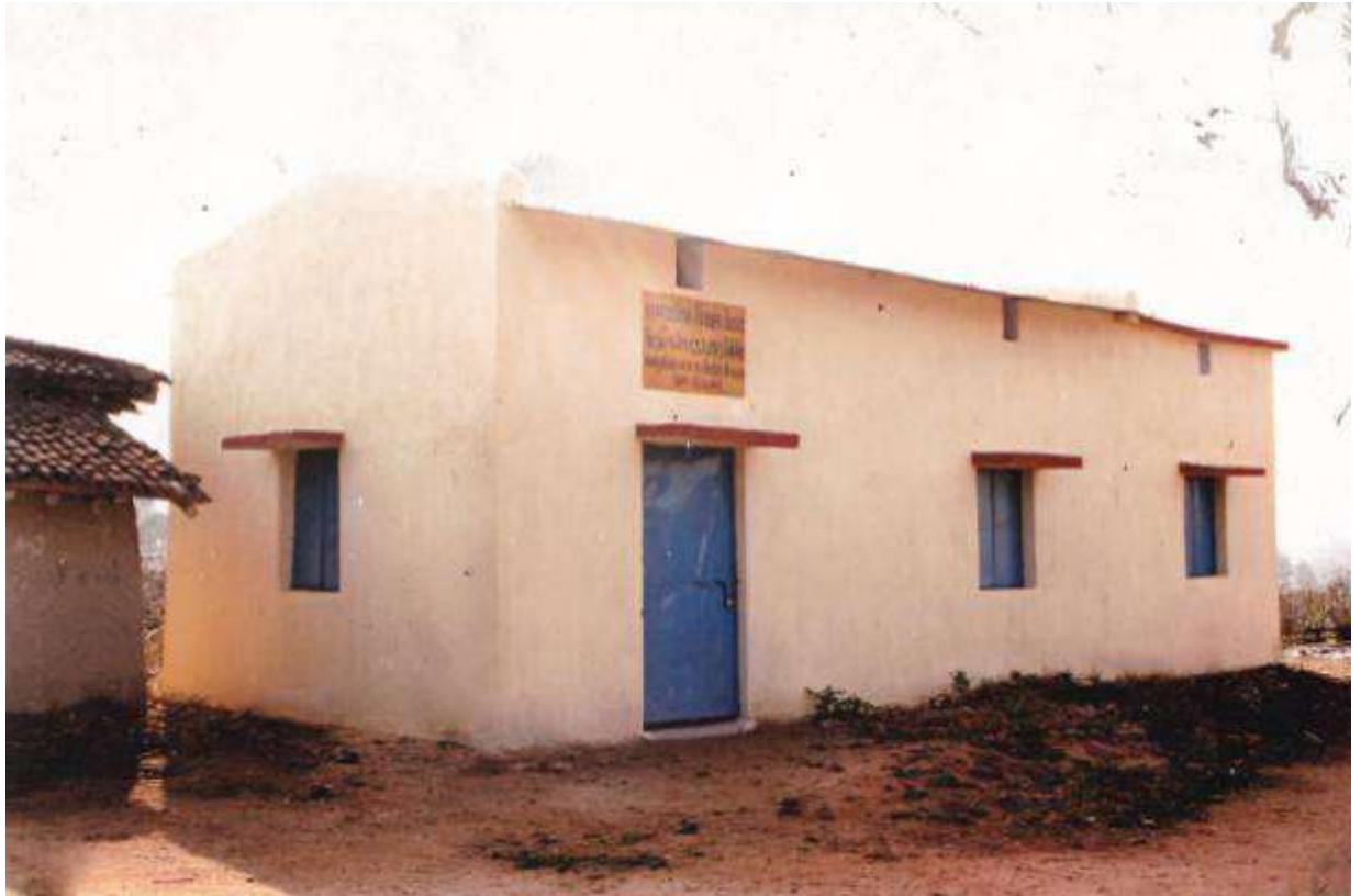
Community hall constructed under CSR scheme of NK Area
