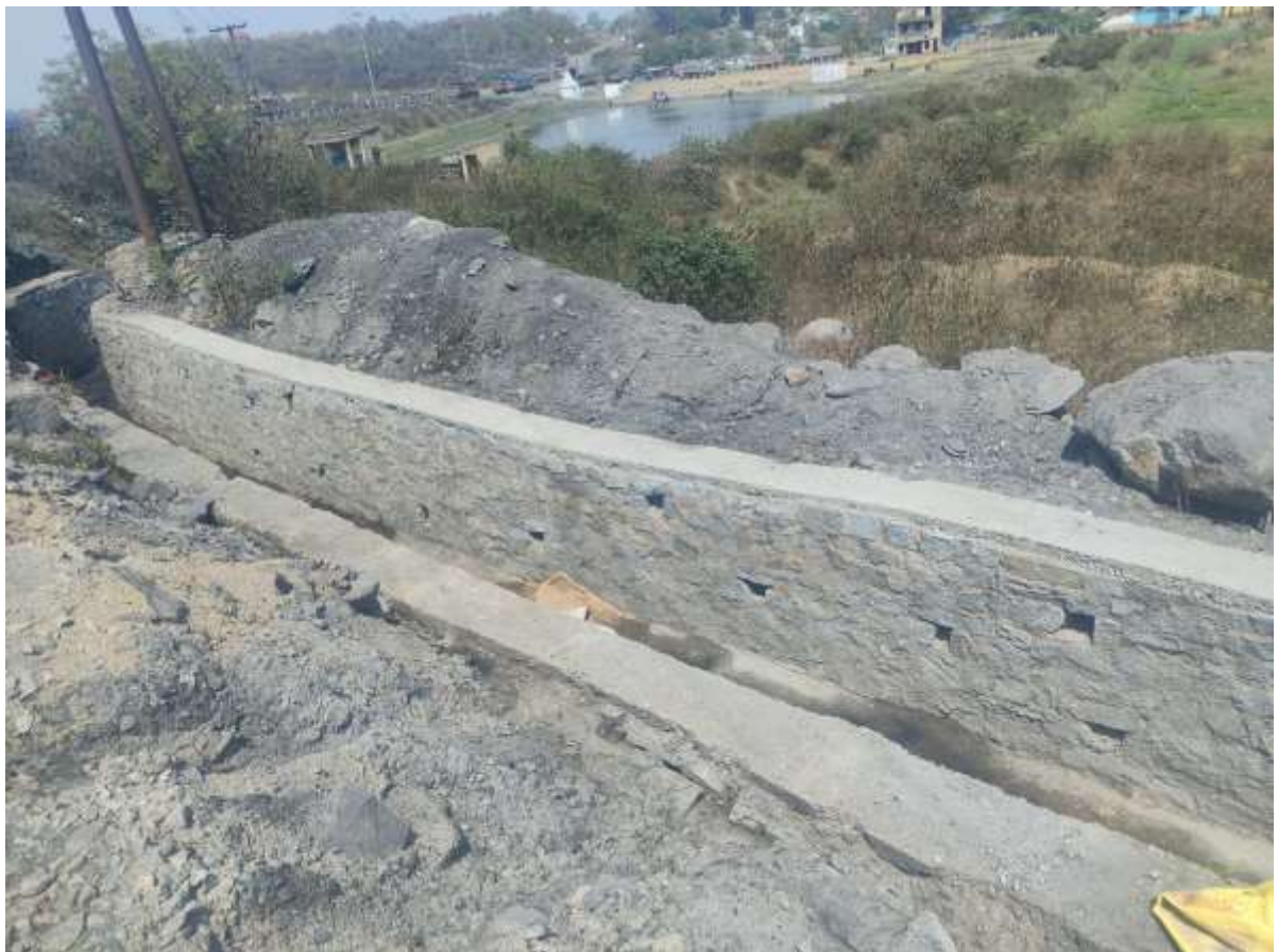
Figure 1.10 Drains in Dakra Siding
