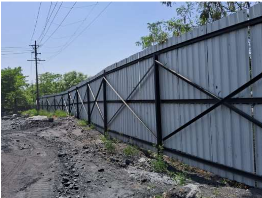
Figure 1.8 Wind breaking Screen with retention walls at Dakra Siding
