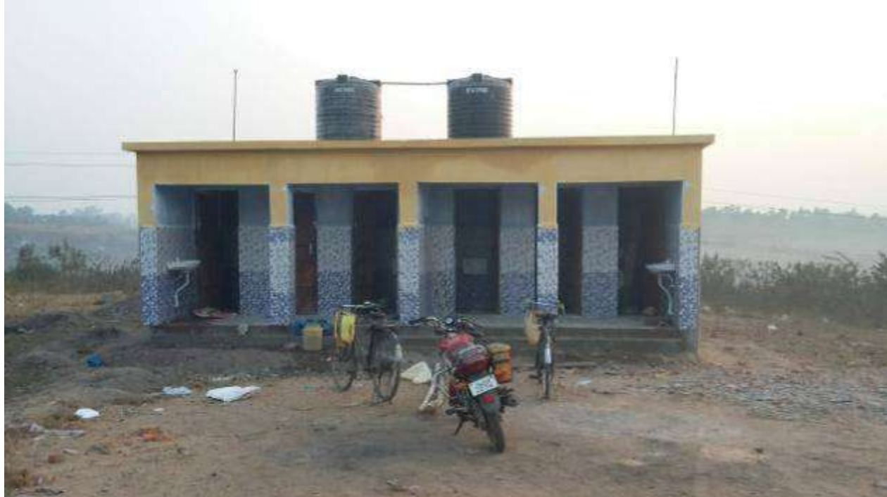
Construction of toilets
