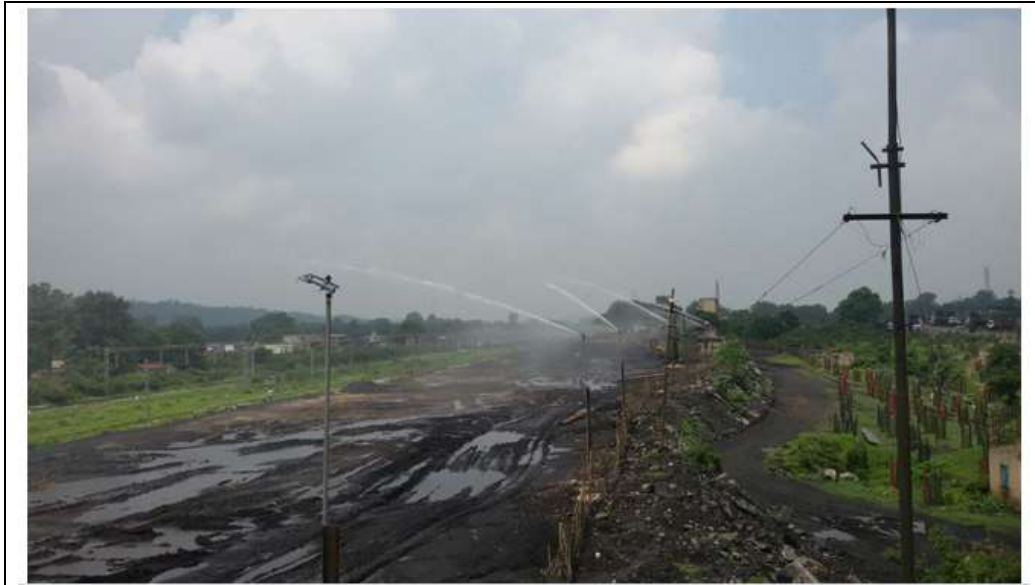
e) Water sprinkler system with plantation (August 2016)
