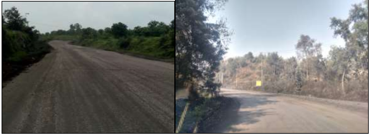
Figure 1.6 3.2 Km approach road
