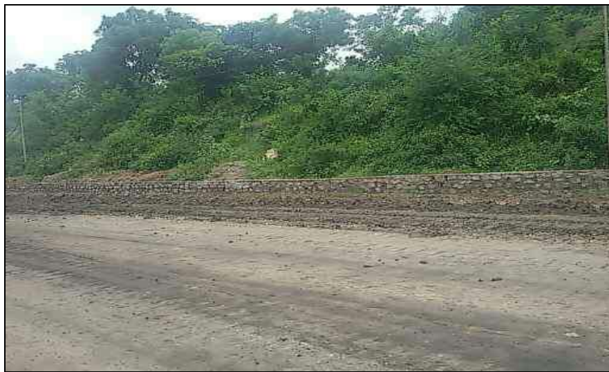
Figure 1.7 Toe wall constructed in Dakra OCP
