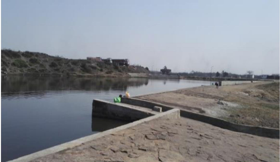
BENTI POND AT ASHOK OC PROJECT, PIPARWAR AREA, CCL.
