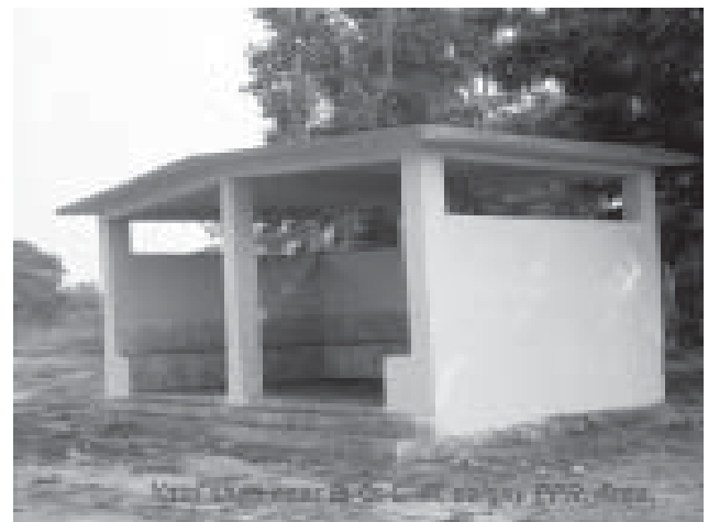
Newly constructed Yatri shed near B.O.C.M Colony, Piparwar Area of CCL
