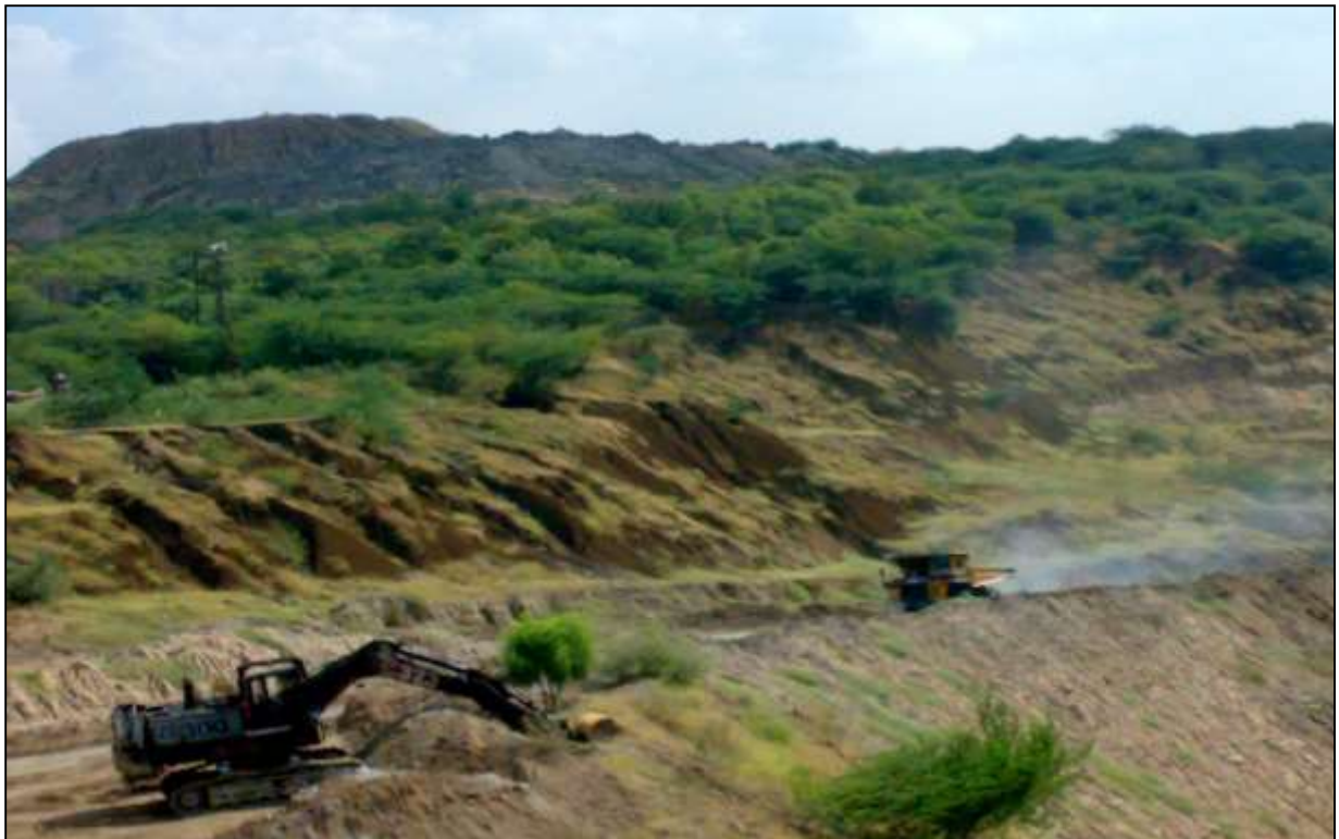
Photograph – 5.6 : Plantation on backfilled area in Pimpalgaon OCP
